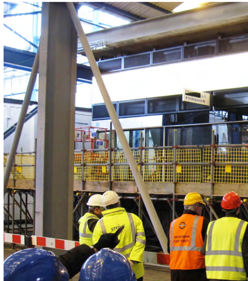
Elizabeth Line running trial for constructability and electrical trials
