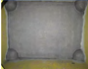
Container After Grit Blasting
